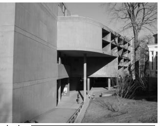
each concrete baffle from north to south, the baffles should admit all sunlight that comes directly from the south.
