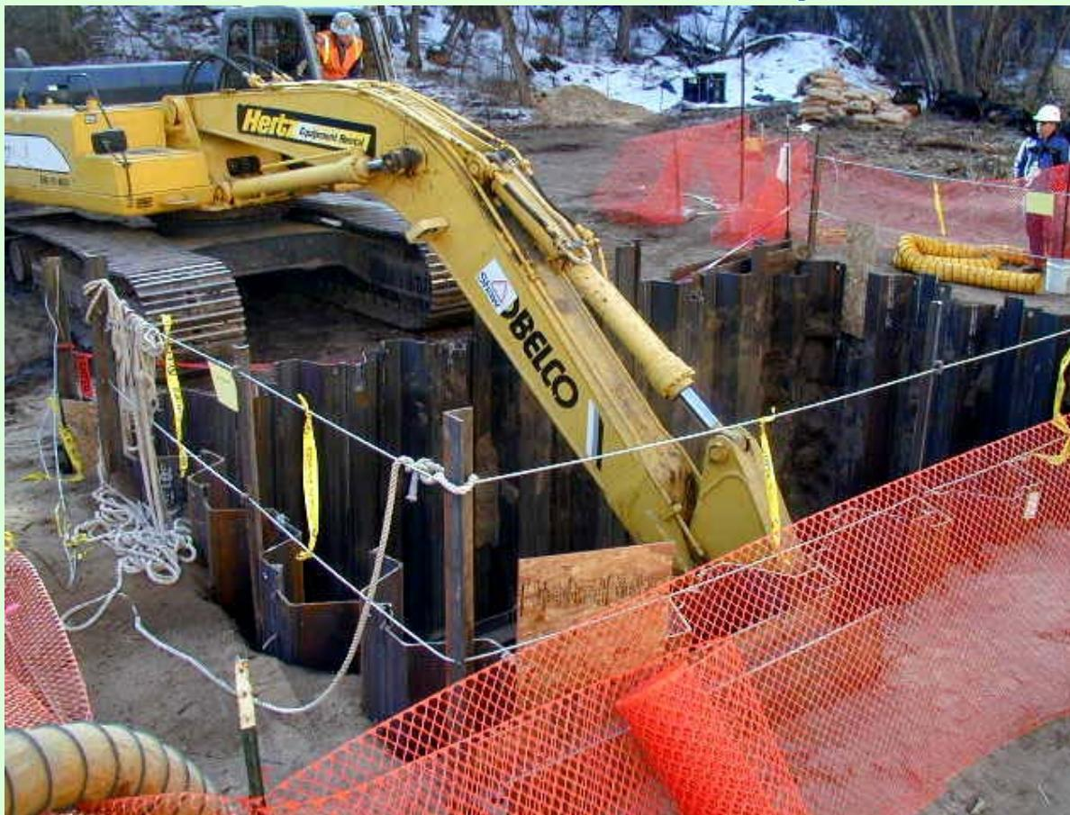
**Crews install a Permeable Reactive Barrier in Mortandad Canyon. The barrier will help control legacy contamination in the canyon by scrubbing shallow groundwater as it moves downstream.**
