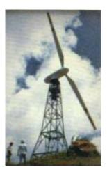
Figure 1: Truss tower supporting the NASA wind turbine generator at Oahu, Hawaii.
